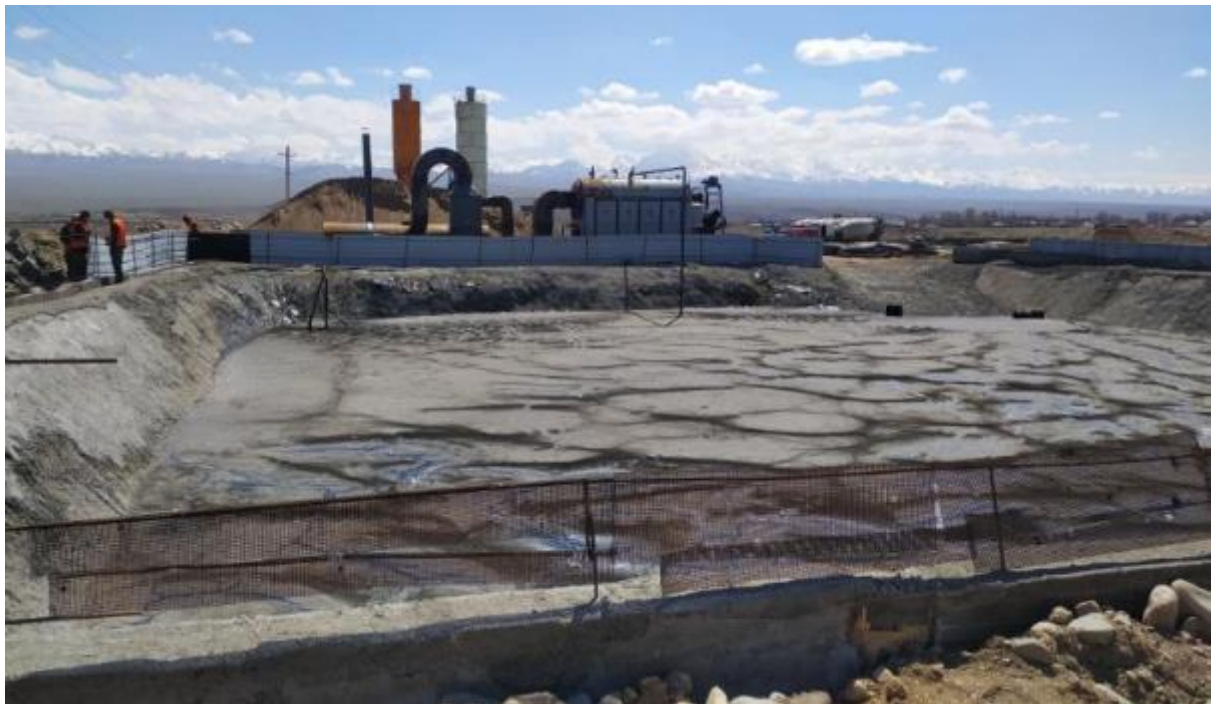
Figure 20: Bitumen pit at the production site (km 148+630).
