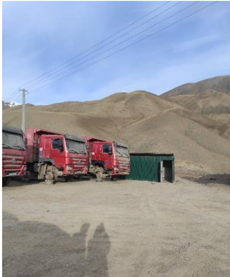
The area of the second construction camp (km 106+300).
