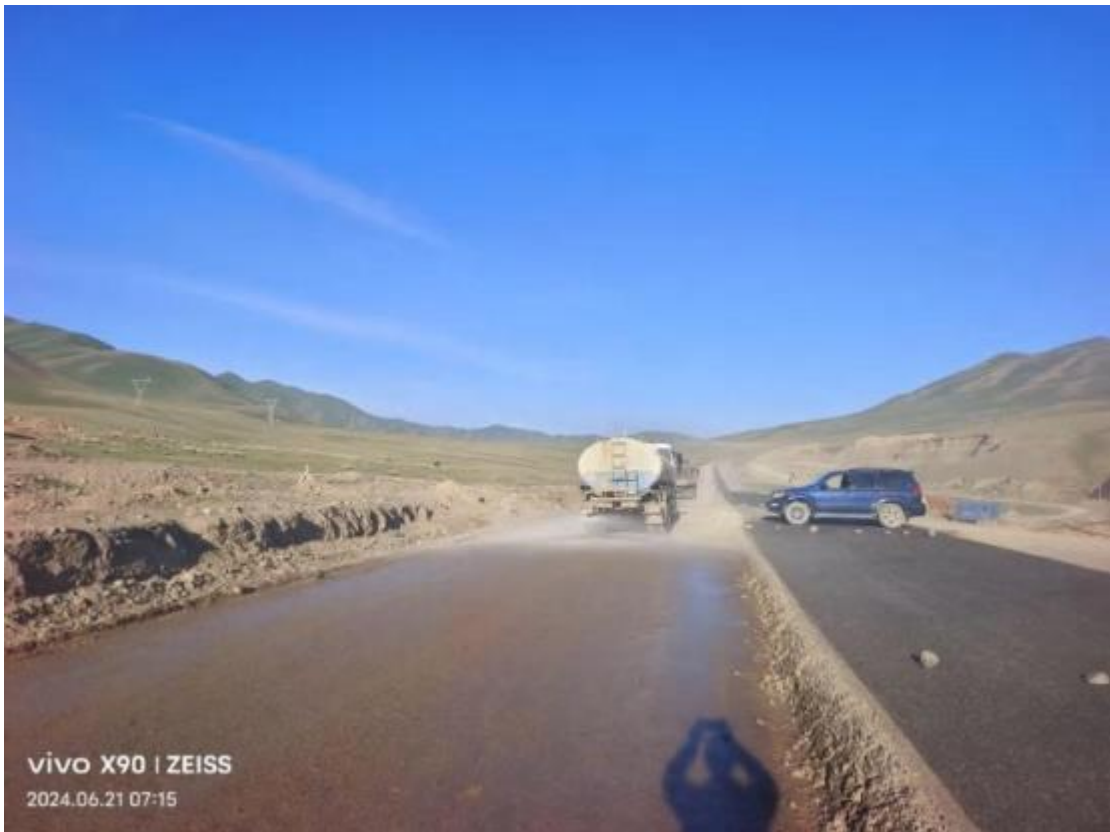
Figure 15: Dust suppression on roads.
