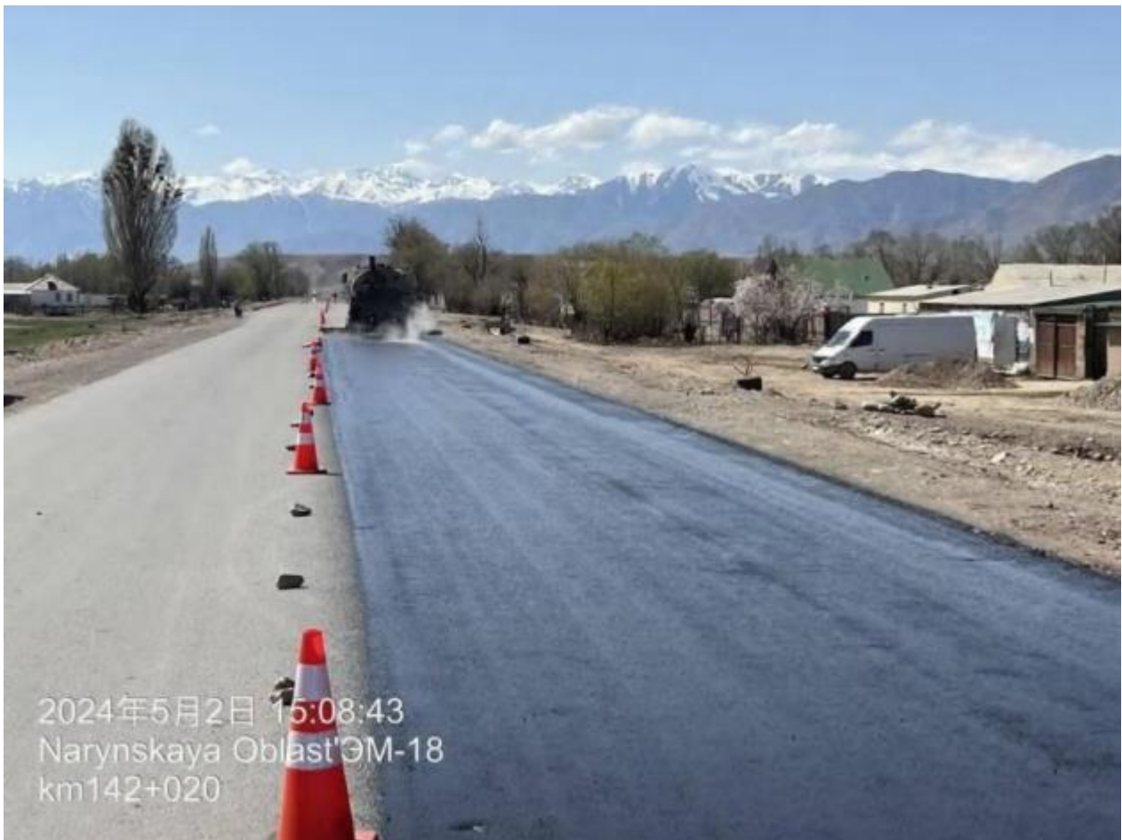
Figure 11: Tack coat, km142+020-km143+020 RHS.
