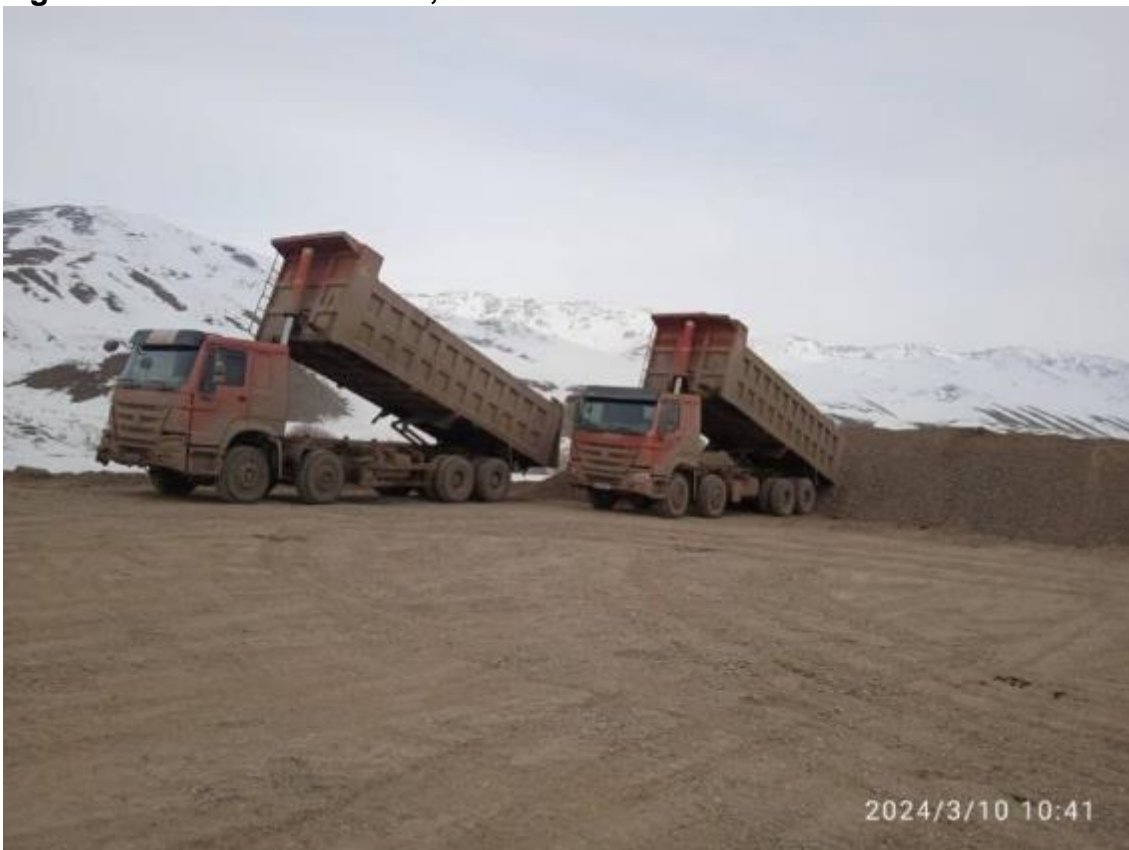
Figure 7: Transfer base material to km122 from km106.
