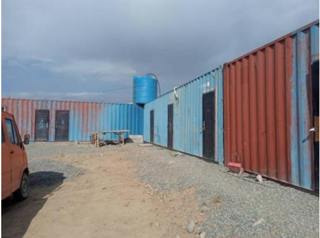
The area of the second construction camp (km 106+300).
