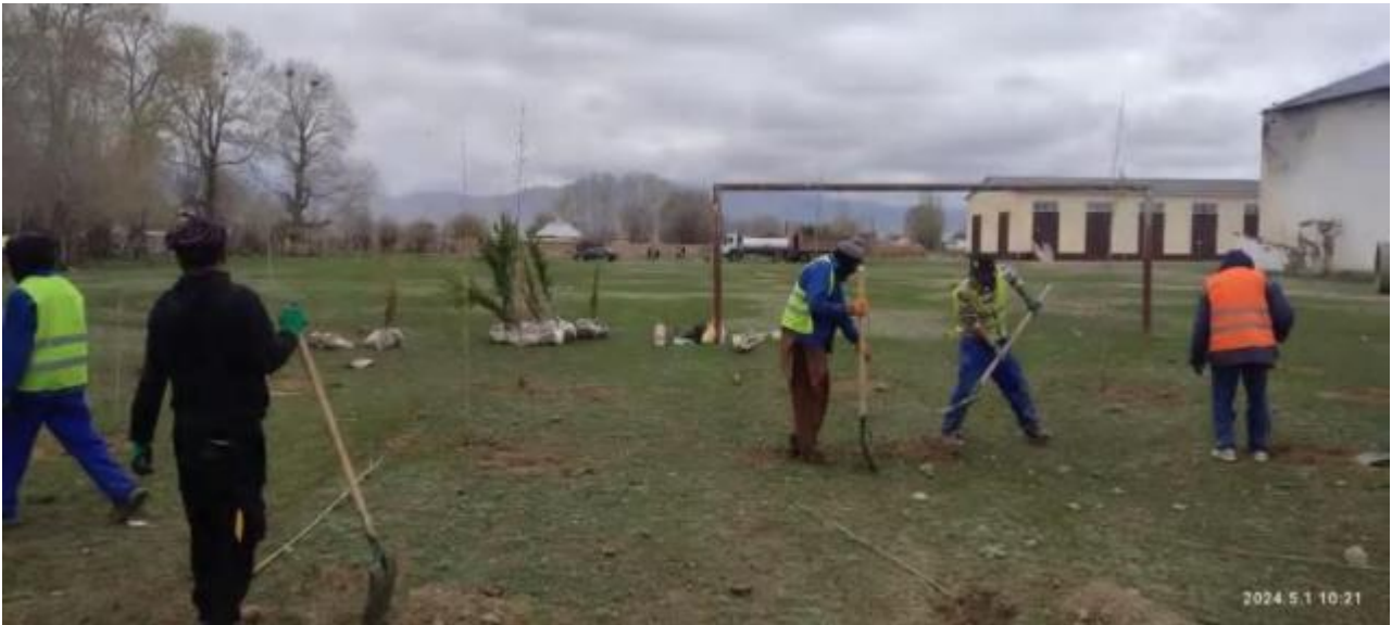
Figure 10: Planting trees, km149+500RHS.
