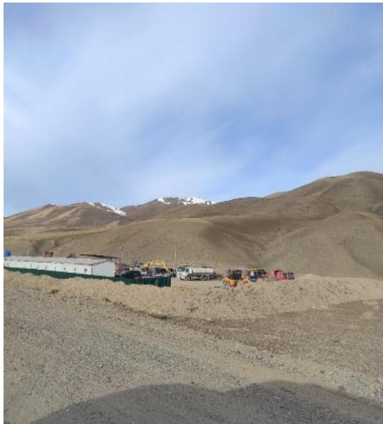
Figure 23: The area of the second construction camp (km 106+300).
