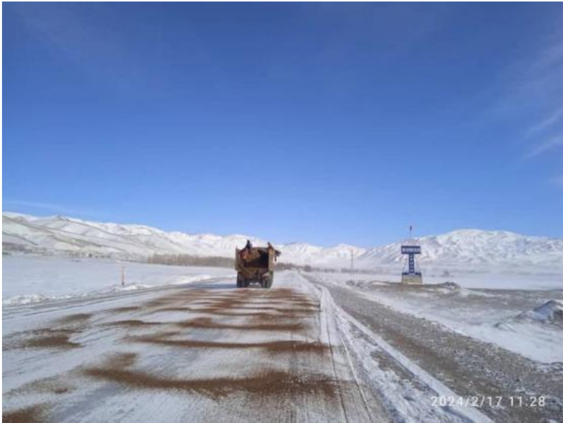
Figure 6: Road maintenance, km 89+500 - km159+200 R&L.
