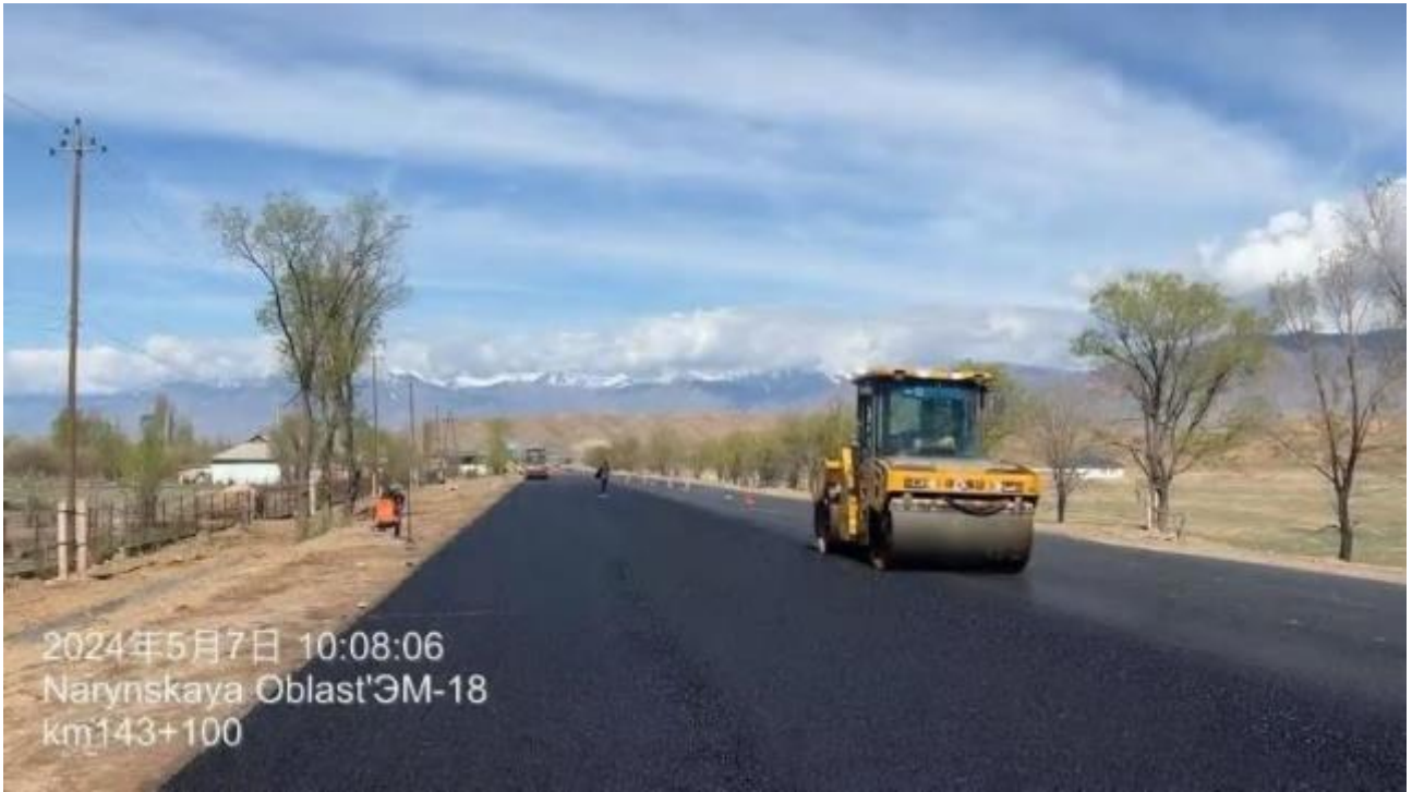
Figure 12: Wearing course, km143+080-km143+300 RHS.
