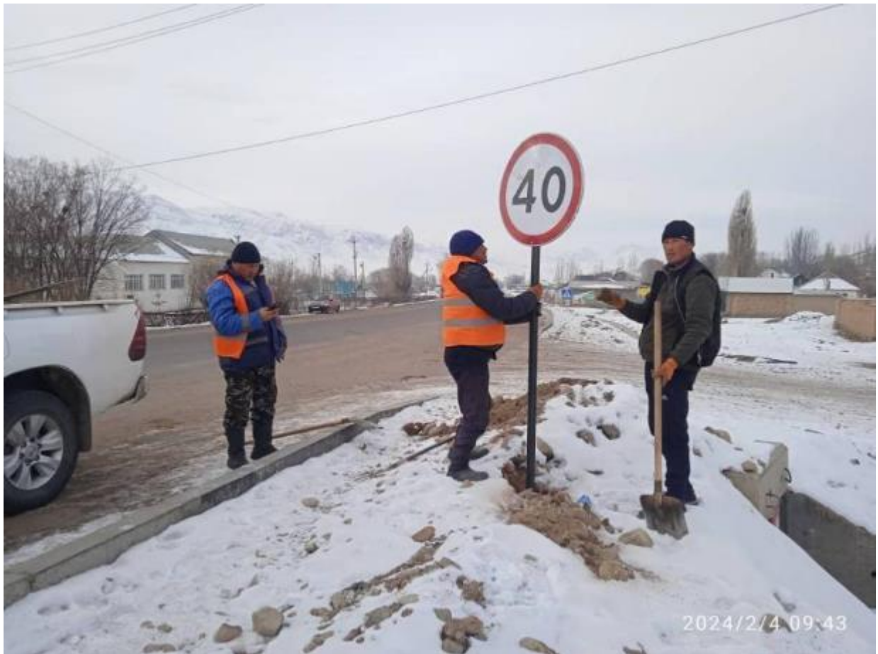
Figure 5: Install temporary signage, km127+650RHS.
