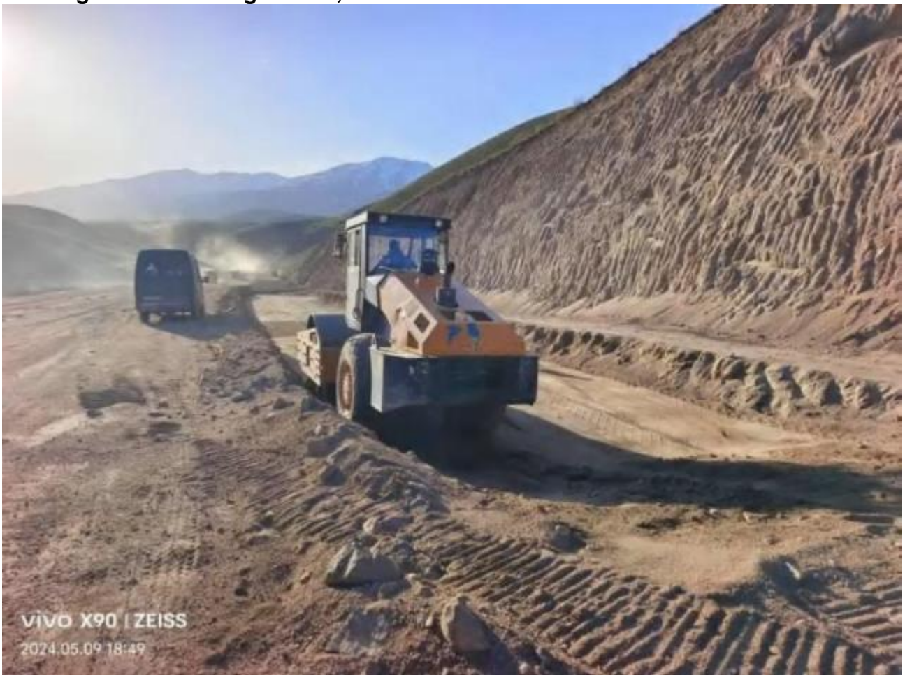
Figure 13: Embankment formation, km 113+600 – km 113+680 RHS.
